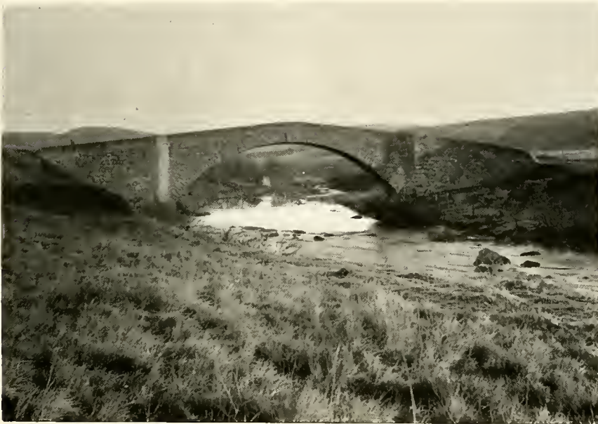
FAILLIE BRIDGE, DAVIOT, INVERNESS-SHIRE.
