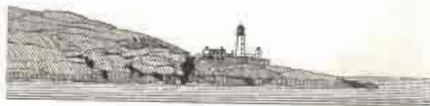
Rob'h Ró lighthouse, bearing 193° (Original dated 1835.)
