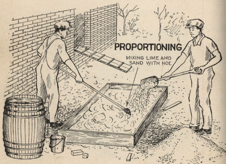
FIG. 3,875.—Preparing lime mortar. Proportioning the sand.
