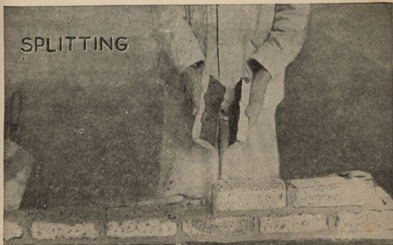
FIG. 4,025.—Appearance of brick after splitting. Showing the kind of split that can be expected.
