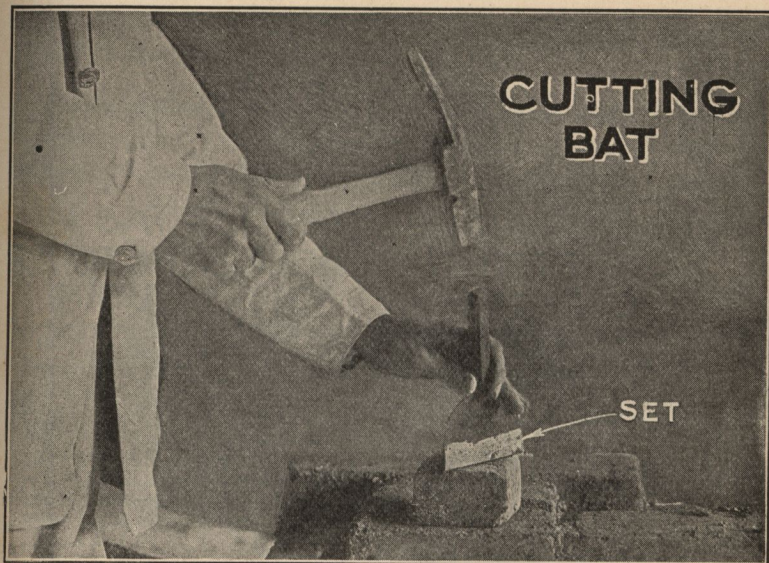
FIG. 4,069.—Bricklayer cutting a half bat with set and hammer. One sharp blow on the set should be sufficient to cause the brick to be broken by one or two sharp flat blows of the hammer on one of the bed surfaces of the brick in line where the line of fracture is desired.
