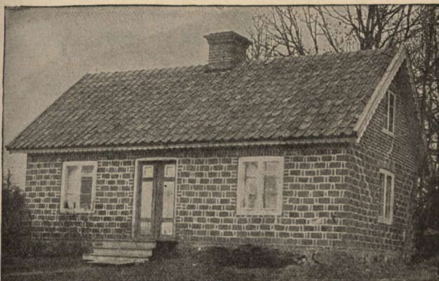
FIG. 4,126.—Bungalow built in 1880 at Arhultemala, Sweden, showing exterior appearance of Ideal wall.
