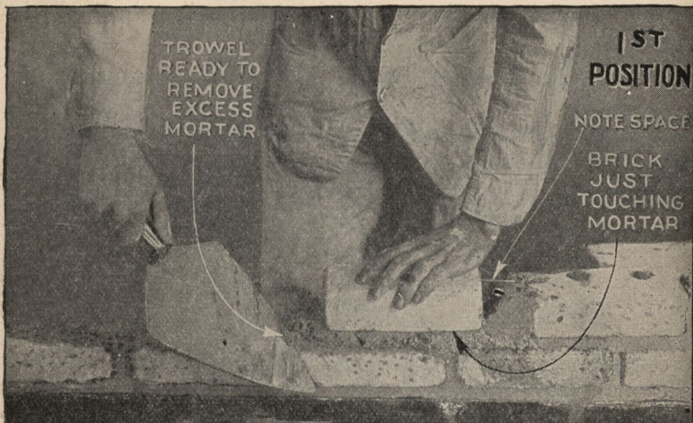
FIG. 3,992.—Brick laying— 1st position . The brick is held in hand with thumb on one side—forefinger on top and other three fingers on other side of brick—palm of hand on brick.
