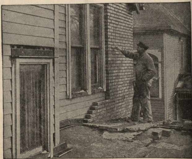
FIG. 4,201.— Brick veneer on old build- ing, II. Ven- eering second story above extension. Note angle irons and work at windows.
