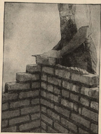
FIG. 4,238.—Bricklayer laying a corner, common bond.
