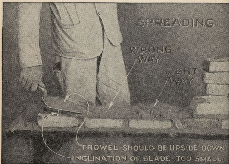
FIG. 3,984.—Spreading mortar, right and wrong way. The trowel should not be held as shown, but should be upside down—that is with back up. Note difference in appearance of mortar laid right and wrong way.
