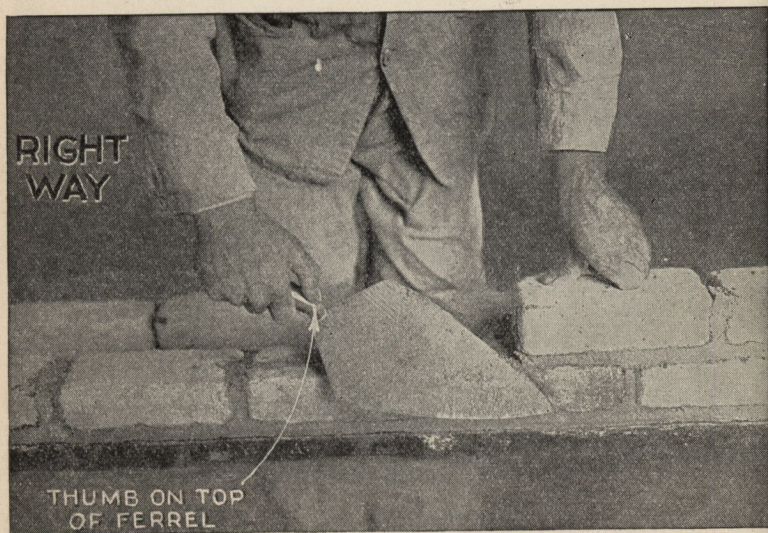
FIG. 3,963.—Holding trowel; right way —thumb on top of ferrel. Note position of thumb on ferrel, in which position the trowel is easily turned as the trowel is moved along the course of brick.
