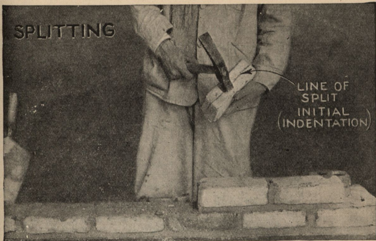
FIG. 4,024.—Splitting brick with head of hammer. The brick should be hammered lightly all around so as to secure a true split.
