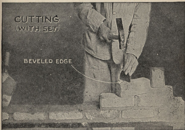
FIG. 4,022.—Method of using a set. The beveled edge on set should be held toward the side being cut off.
