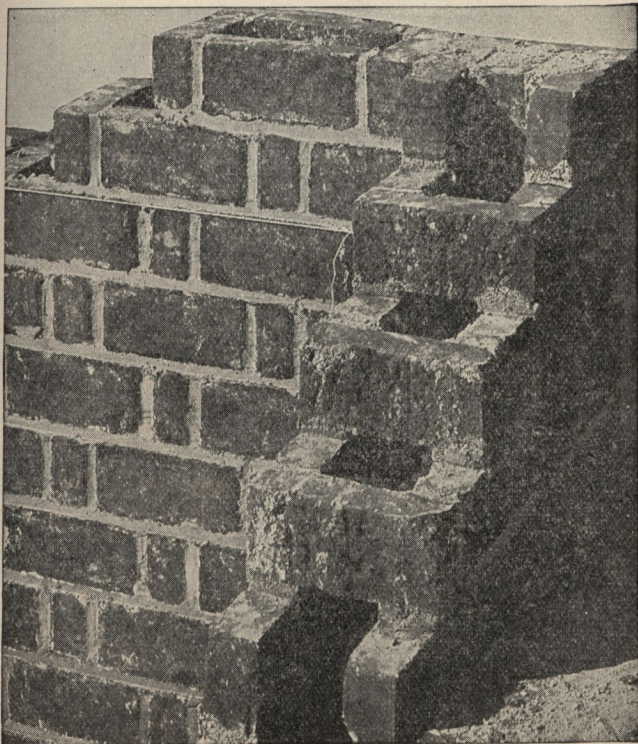
FIG. 4,124.—Corner construction of Ideal all rolok wall showing 2\frac{1}{4} in. webs and ventilated air space.
