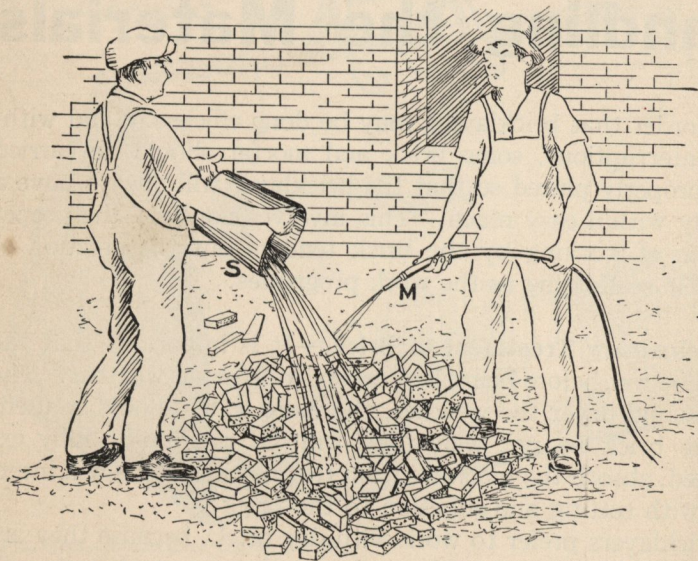
FIG. 3,952.—Two methods of wetting the brick: 1, with hose from hydrant, as at M ; 2, with pail of water, as at S .
