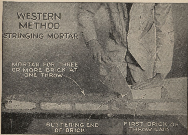
FIG. 3,999.—Western method or method of laying mortar for several brick at one throw. Mortar is thrown for 3 to 5 brick, depending on the kind of brick and consistency of mortar.
