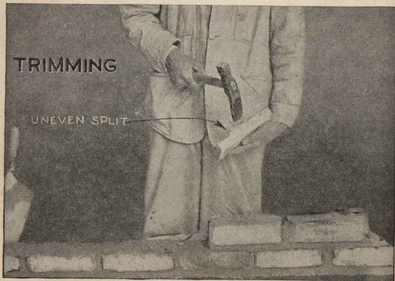
FIG. 4,028.—Trimming with peen of hammer. Should be done with short sharp blows.
