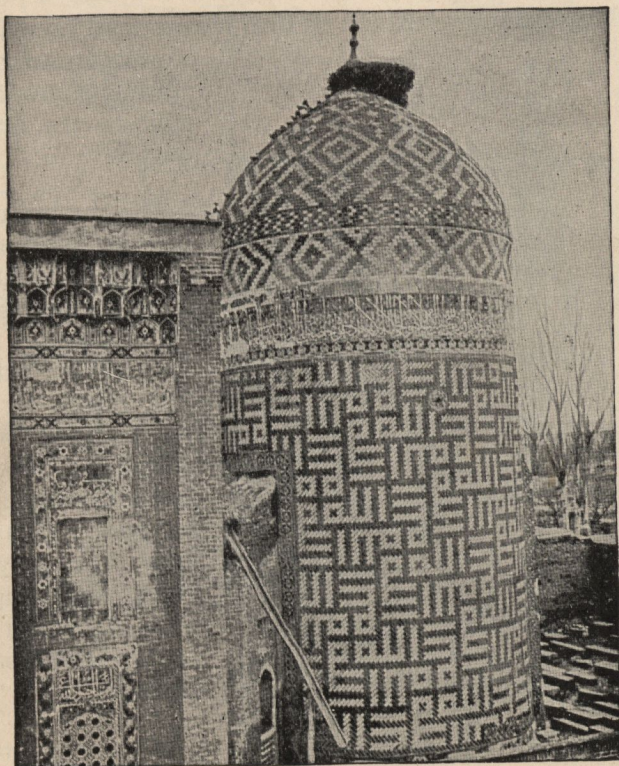
FIG. 3.774.—Brickwork in old Persian tomb at Ardabil.
