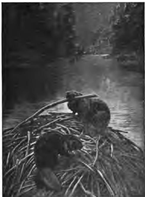
BUILDING A DAM
