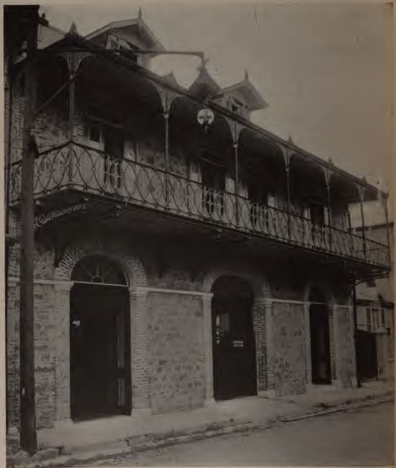
RUST, TROWBRIDGE & CO., CHACON STREET
