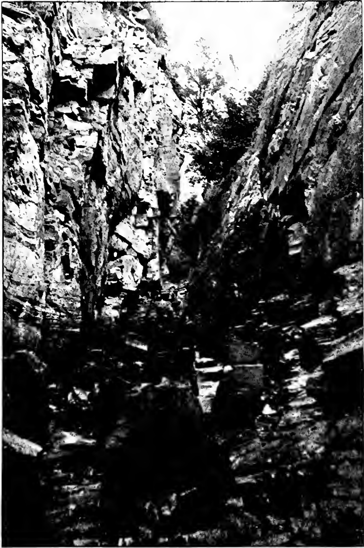
THE INVERMORISTON PASS, FROM BOTTOM OF CUTTING (WATER TURNED OFF).
