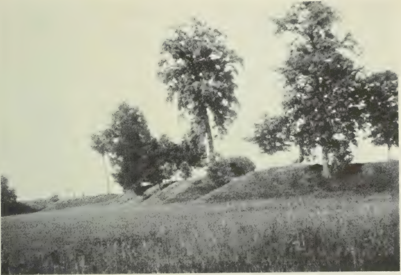
2. EAST WALL OF FORT ANCIENT, WARREN COUNTY
