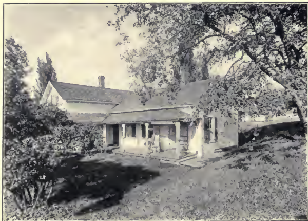
THE VERANDA WHERE STEVENSON WALKED AND DREAMED
