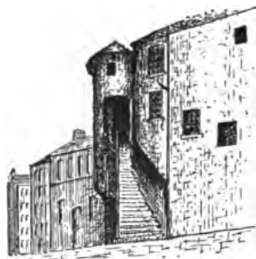
QUAINT HOUSE IN BURNET'S CLOSE.
