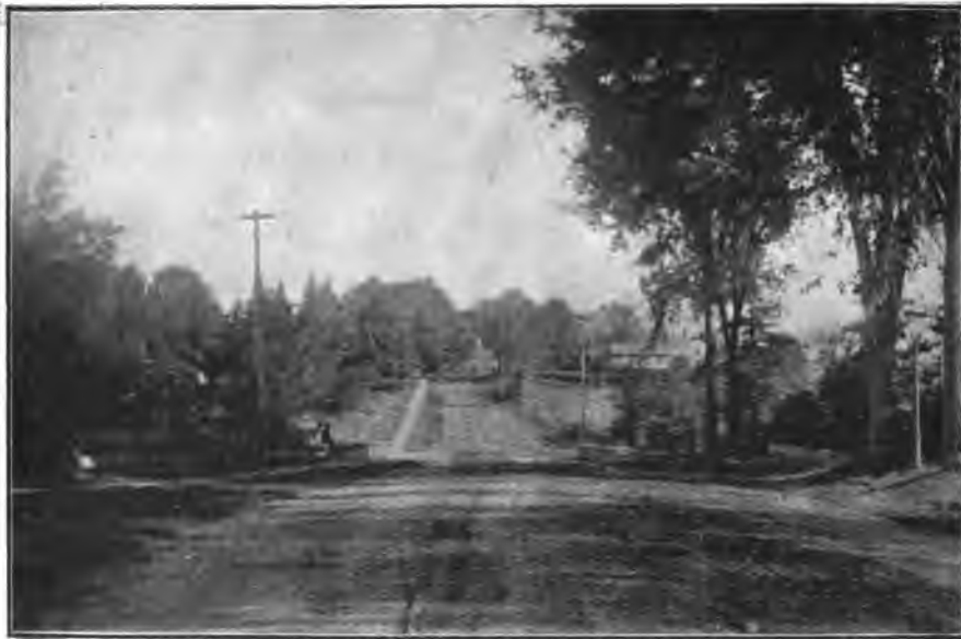
ROADWAY LEADING INTO MAIN STREET, ARGYLE, NEW YORK STATE.
