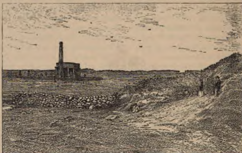
HILLSD, SHOWING THE FIRST WATER TANK.
