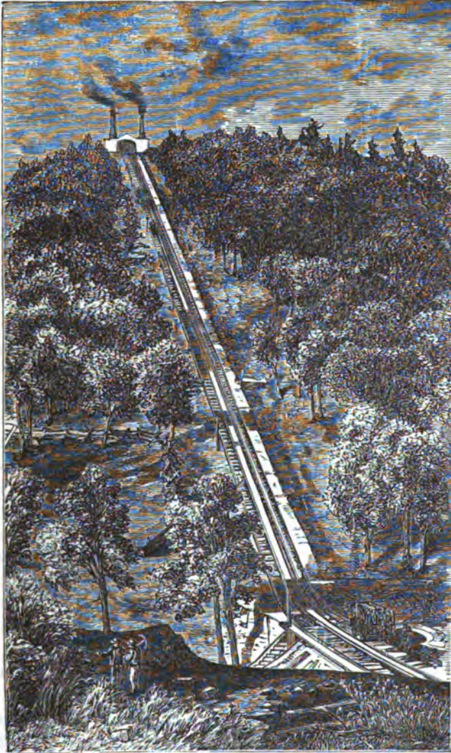
MOUNT PISGAH INCLINED PLANE AT MAUCH CHUNK, PA.— Built in 1826, being, with its gravity railroad, and several other connecting planes, at that time, the longest railroad in the United States, and the first, except that at Quincy, Mass., which was completed two months earlier. This "Switch-Back" Railroad, as it is called, has been superseded by a tunnel at Nesquehoning, and is now only used for excursions.
