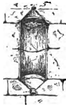
THE LAMP NICHE, CORSTORPHINE CHURCH.
