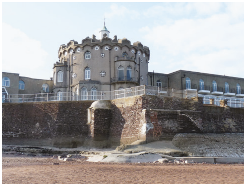
Figure 13.13 The Central Rotunda, Redcliffe Towers, Paignton, Devon, with the door of the plunge-pool tunnel opening above the beach. Photograph by Diane James © 2013.
