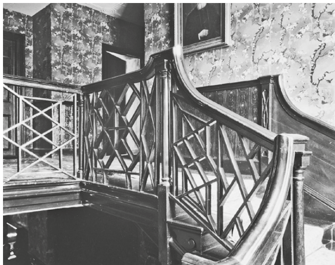
Figure 14.2 The 'Chinese' staircase at Bishopsgate House, showing the first floor landing. The stylized wave design carved into the tread ends is just visible in the bottom centre of this image. DI2011_1011, NPRN 15946. © Crown copyright: Royal Commission on the Ancient and Historical Monuments of Wales.
