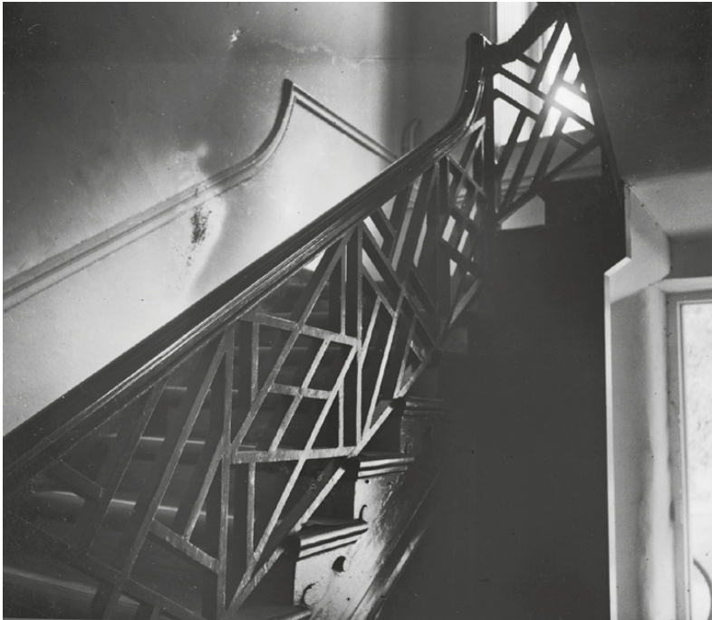
Figure 14.1 The main staircase from the entrance hall at Tan-yr-Allt, showing the ascent to the first floor and hinting at fluted window reveals. DI2013_0674, NPRN 16895. © Crown copyright: Royal Commission on the Ancient and Historical Monuments of Wales.
