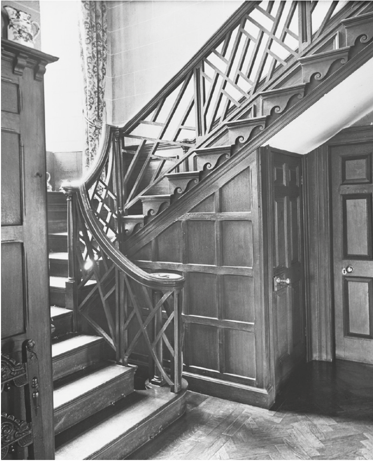
Figure 14.3 The ‘Chinese’ staircase at Trefeilir, probably photographed in the 1930s, showing the main balustrade of the staircase with its latticework. DI2011_1010, NPRN 15898. © Crown copyright: Royal Commission on the Ancient and Historical Monuments of Wales.
