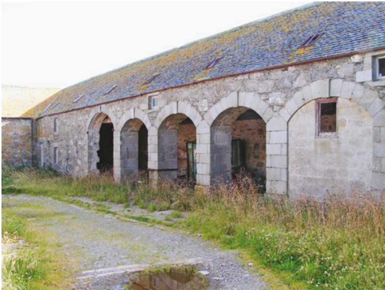
Figure 16.3 Cart arches, Mains of Carnousie. Image courtesy of Alistair Mutch.
