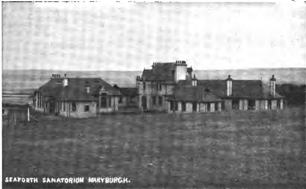
THE SEAFORTH SANATORIUM—BACK VIEW.
