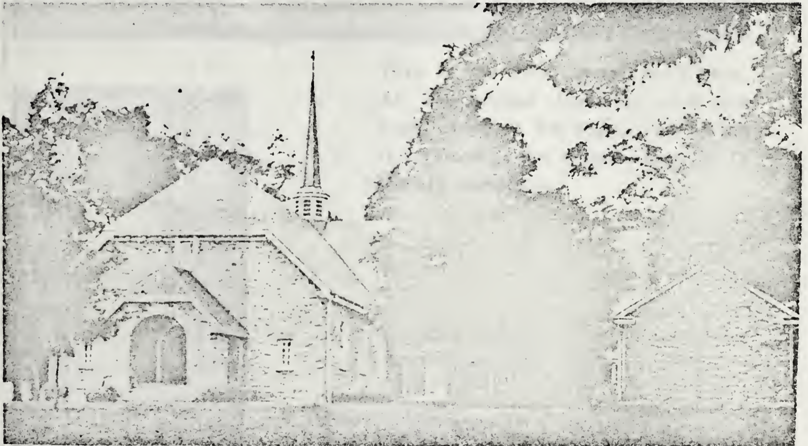
Old Stone Church as it is today. The back of the old church was taken out. The walls were extended and arms, as of a cross, were added. To the right Sunday School rooms were then built. The small stone building in the foreground is the Retiring House. It is not the original one which stood close against the middle window which was then a door behind the pulpit, but this one was built in 1847.
