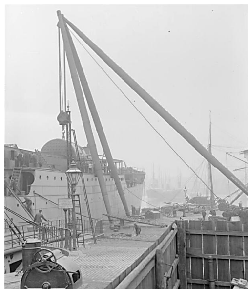
80-ton Shear Poles , lifting boiler onboard a vessel, pre-1910.
