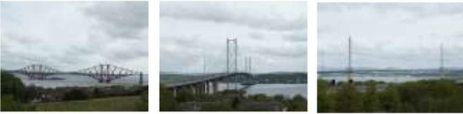
The 3rd Bridge the Queensferry Crossing was built to take the ever-increasing traffic flow; the old bridge was designed for 11 million vehicles per year and by 2006 was dealing with traffic of 23 million vehicles per year. The Queensferry Crossing is a 3 tower Cable-Stayed Bridge with an overall length of 2.7 km. The old 2nd bridge the Forth Road Bridge is now being used for commuter traffic IE. Buses and taxis.
