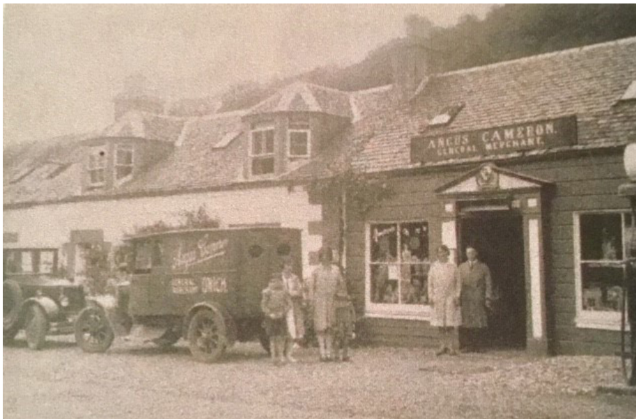
The Cameron Family outside The Stores at Onich, 1925
