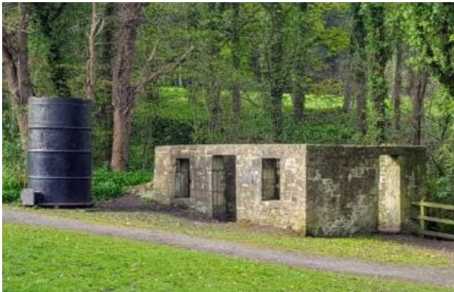
James Watt Cottage/Workshop, Kinneil
