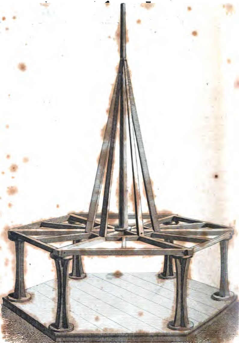
Cast-Iron Pillar Corn Stands, with a Top made of Timber.
