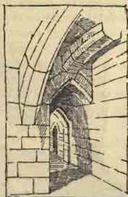
FIG. 456a.—Crookston Castle. Springing of End Rib.
