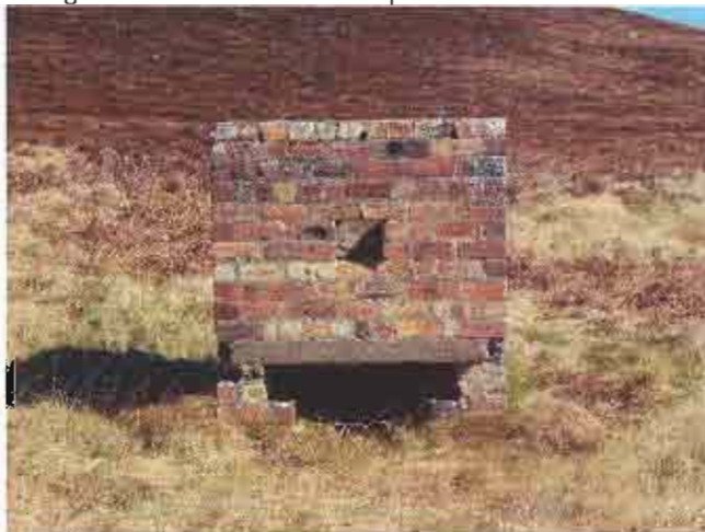
And 2.) The brick structures that served to hold the fires that generated the heat to keep the structures warm.
