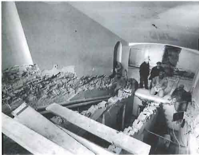
February 23, 1950: Workers remove the main staircase.
