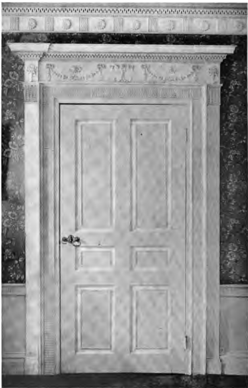
PLATE CV.—Detail of Doorway, East Parlor, Pierce-Johonnot-Nichols House.
