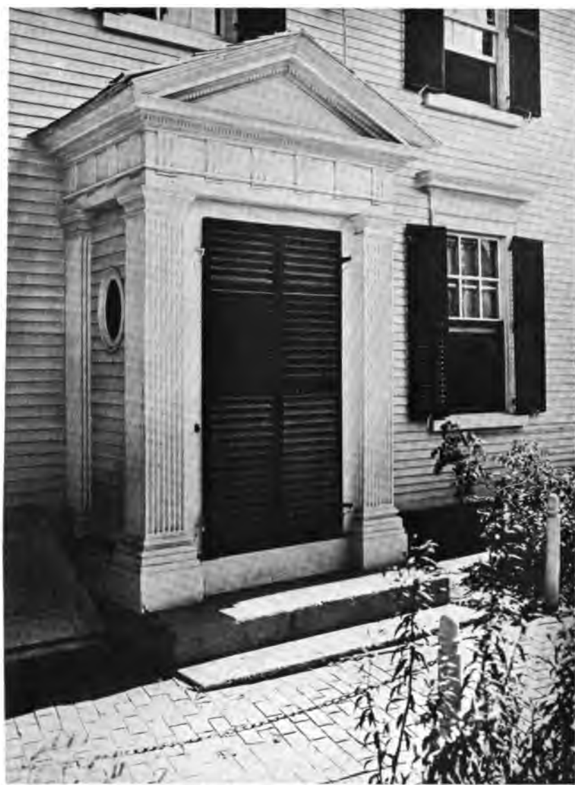
PLATE XCII.—Enclosed Side Porch, Pierce-Johonnot-Nichols House.
