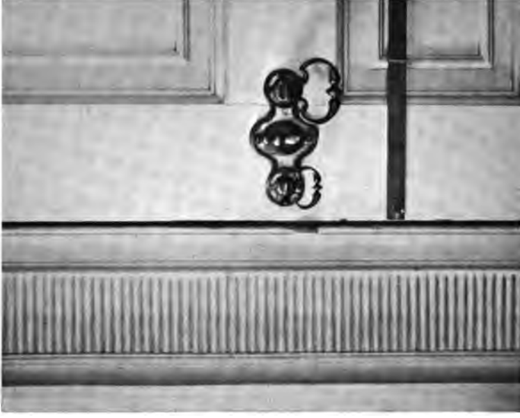
PLATE XXXIII.—Dado, Surbase, Baseboard, and Architrave Casing, Pierce-Johonnot-Nichols House; Door Paneling, Casing, and Drop Handle.
