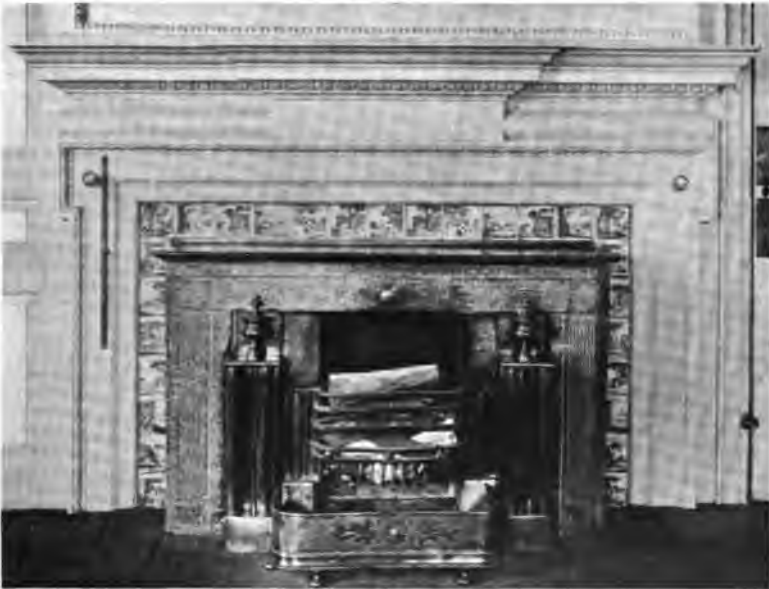
PLATE C.—Embrasured Windows and Seats, West Parlor, Pierce-Johonnot-Nichols House; Detail of Mantel.
