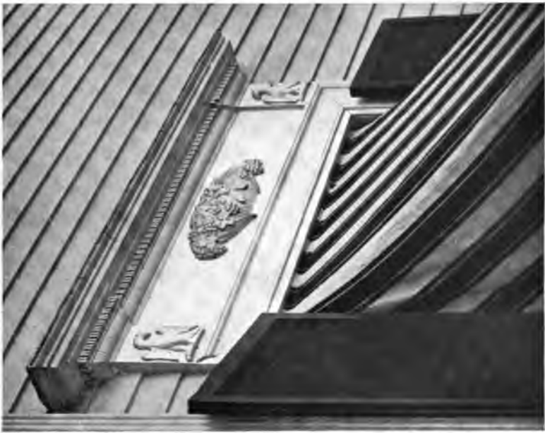
PLATE XVII.—Keyed Marble Lintel, Peabody-Siltsbee House; Entablature of Window Frame, "Oak Hill."
