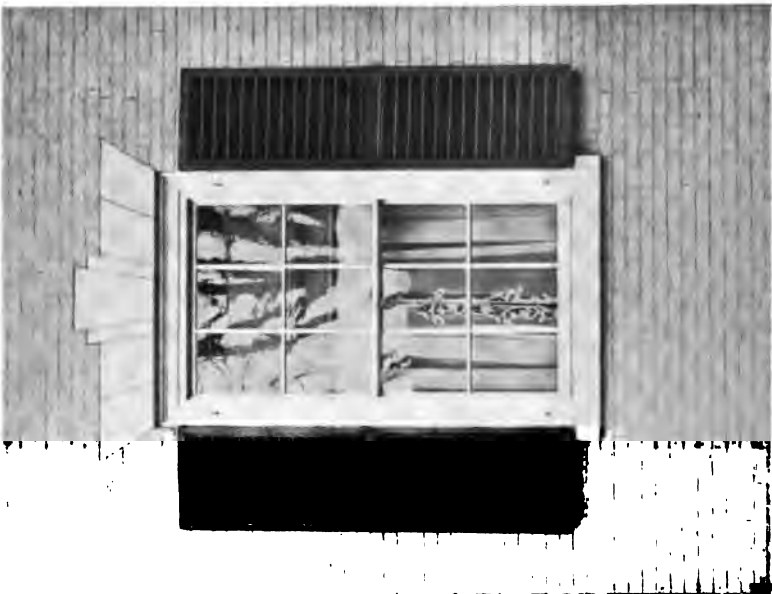
PLATE XVII.—Keyed Marble Lintel, Peabody-Siltsbee House; Entablature of Window Frame, "Oak Hill."
