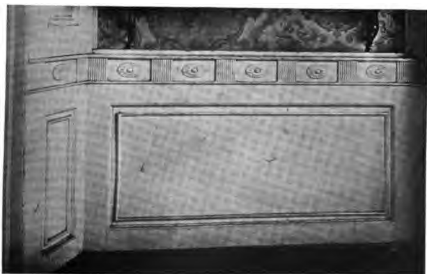
PLATE XXXII.—Stucco Cornice in Derby-Crowninshield-Rogers House; Wainscot and Surbase.
