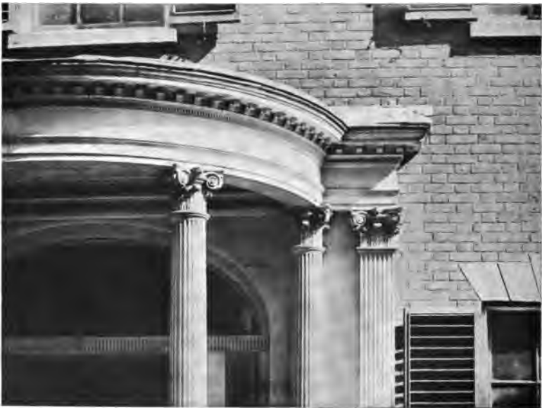
PLATE XXV.—Tucker-Rice House, erected in 1800; Detail of Porch.
