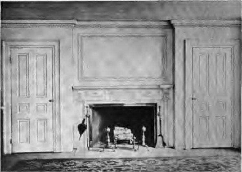
PLATE CXI.—East Front Chamber, Pierce-Johonnot-Nichols House; Architectural Treatment of Rear Wall.
