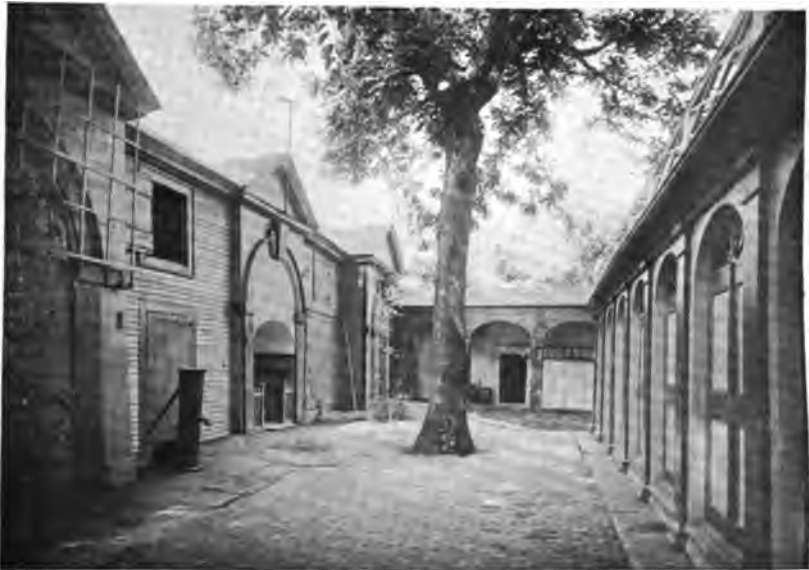
PLATE XCIV.—Paved Courtyard between Pierce-Johonnot-Nichols House and Barn, from two viewpoints.
