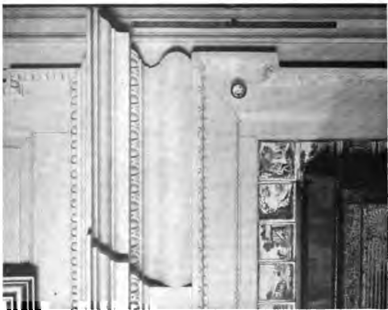
PLATE CI.—Detail of Chimney Piece and China Closet, West Parlor, Pierce-Johonnot-Nichols House; Corner Section of the Mantel.
