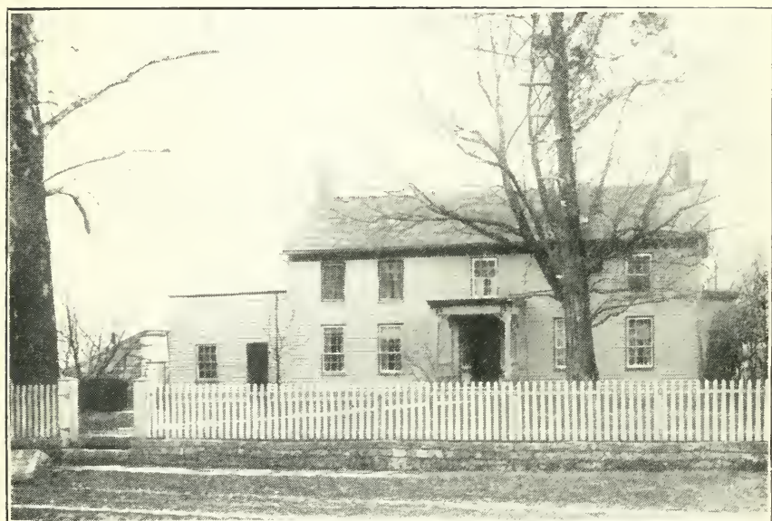
The Dunn Homestead, Jefferson County, Indiana. Built 1809.
