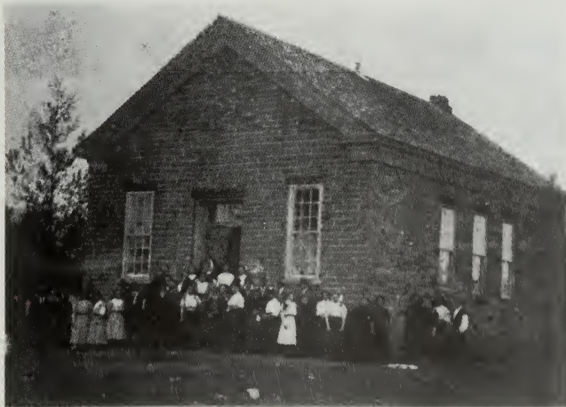
The Sleepy Hollow School, one of Heber's early school buildings.
