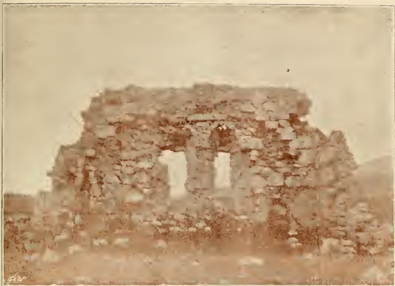
RUINED GABLE OF ST MARY'S CHURCH, HOWMORE, SOUTH UIST.
