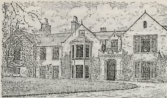
BRACO HOUSE (REBUILT AND MODERNISED)
