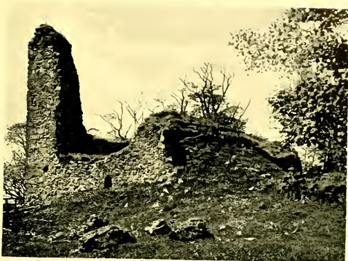
LOCHWOOD TOWER, DUMFRIES.
