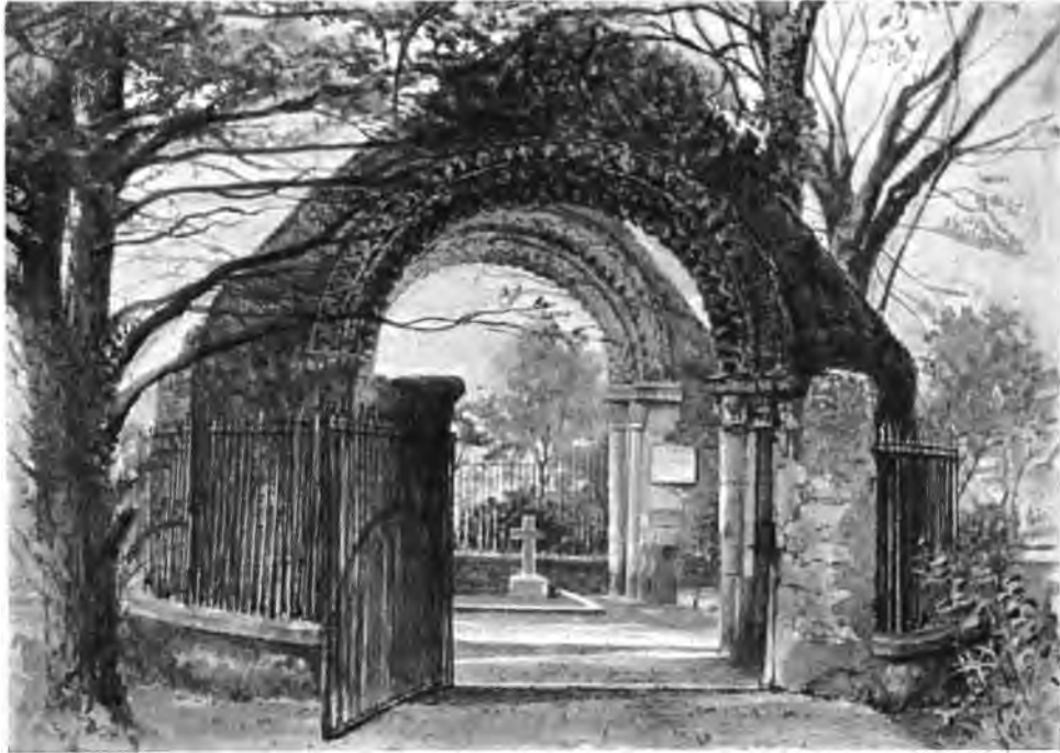
RUINS OF ST. BALDRED'S CHURCH, TYNINGHAME.
