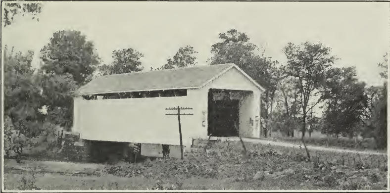
Covered Bridge Over Coal Creek
