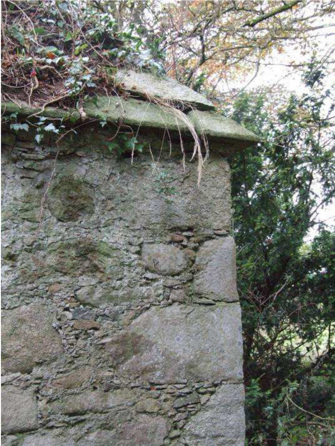
St Medden's Kirk stone tiled roof.
