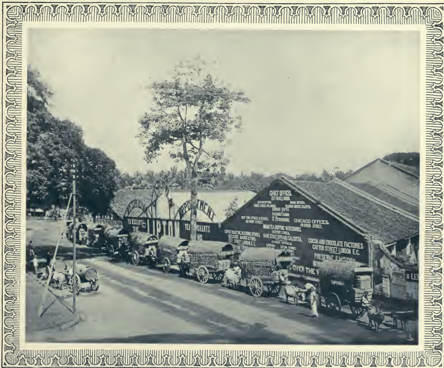
Lipton's Shipping Warehouse, Colombo.
