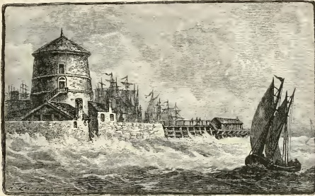
SIGNAL TOWER, LEITH PIER, 1775. (After Clerk of Eldin.)
