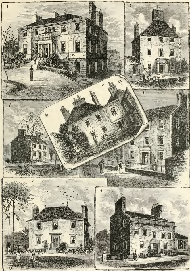
1, BONNINGTON HOUSE; 2, STEWARTFIELD; 3, REDBRAES; 4, SILVERMILLS HOUSE; 5, BROUGHTON HALL; 6, POWDER HALL; 7, CANONHILLS HOUSE.
