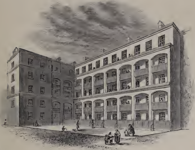
SOUTH AND WEST SIDE OF INTERNAL QUADRANGLE TO MODEL HOUSES, STREATHAM-STREET, THE ENCLOSURE WALL ON THE EAST SIDE BEING REMOVED.
