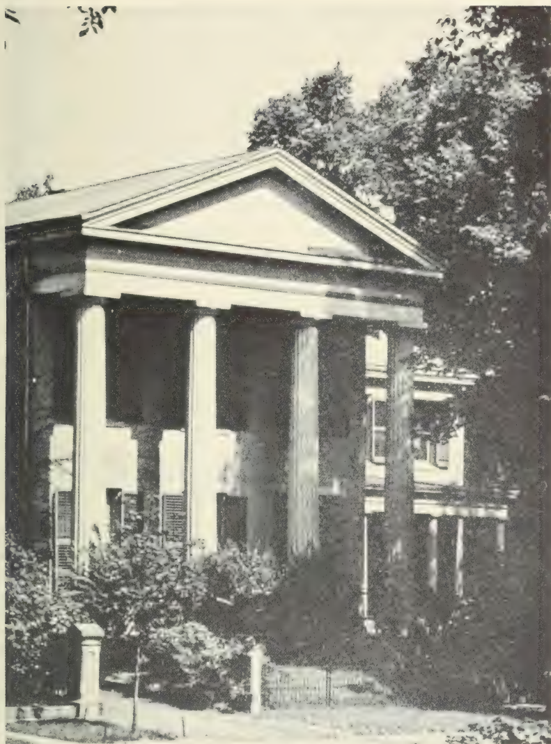
3. HOME AT CHILLICOTHE ERECTED IN 1840 An example of the Classical Revival. Courtesy of Frank J. Roos, Jr.
