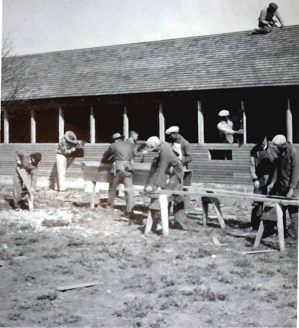
NEW CONSTRUCTION BY STUDENT CARPENTERS
