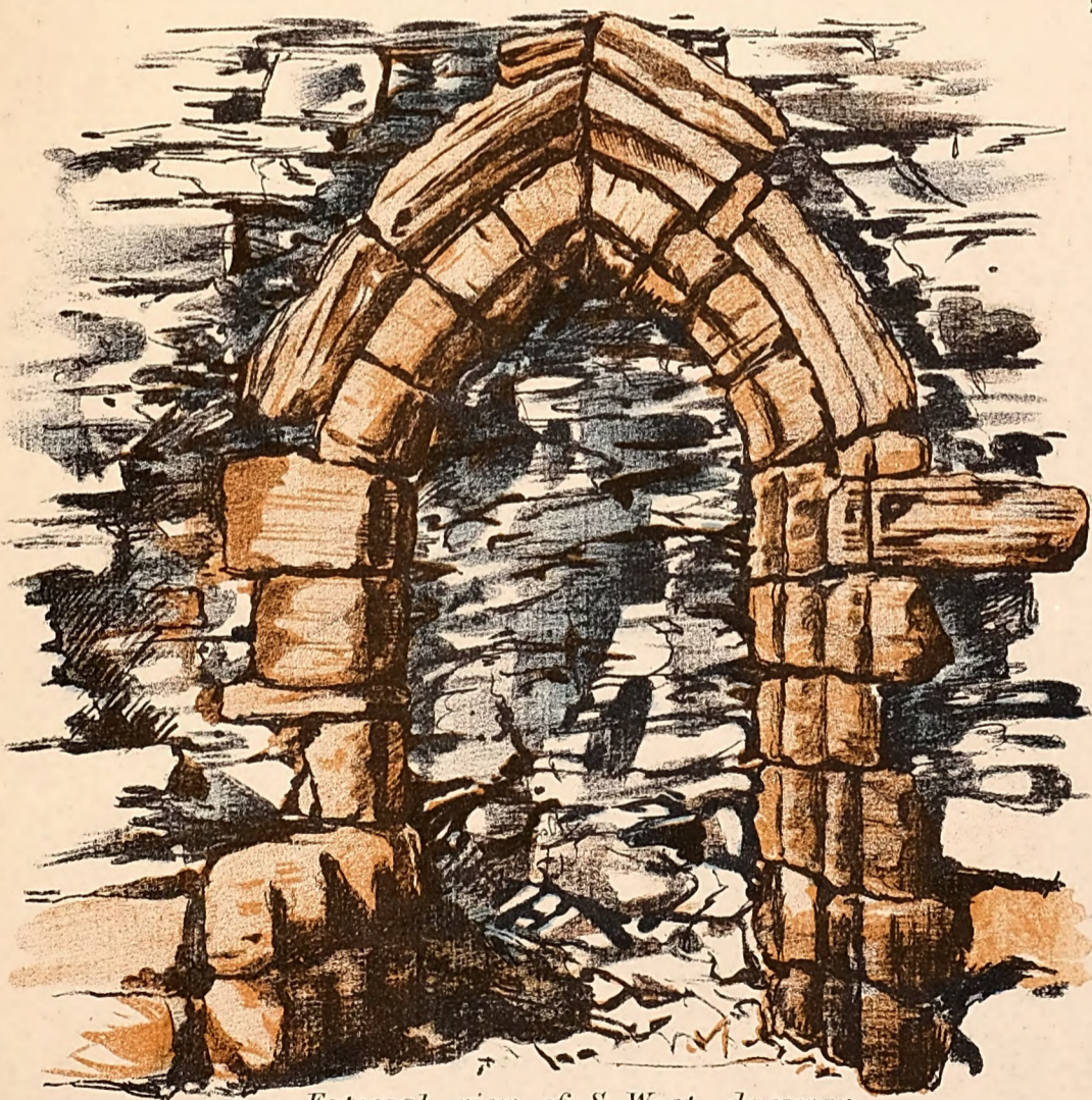
External view of S. West doorway
